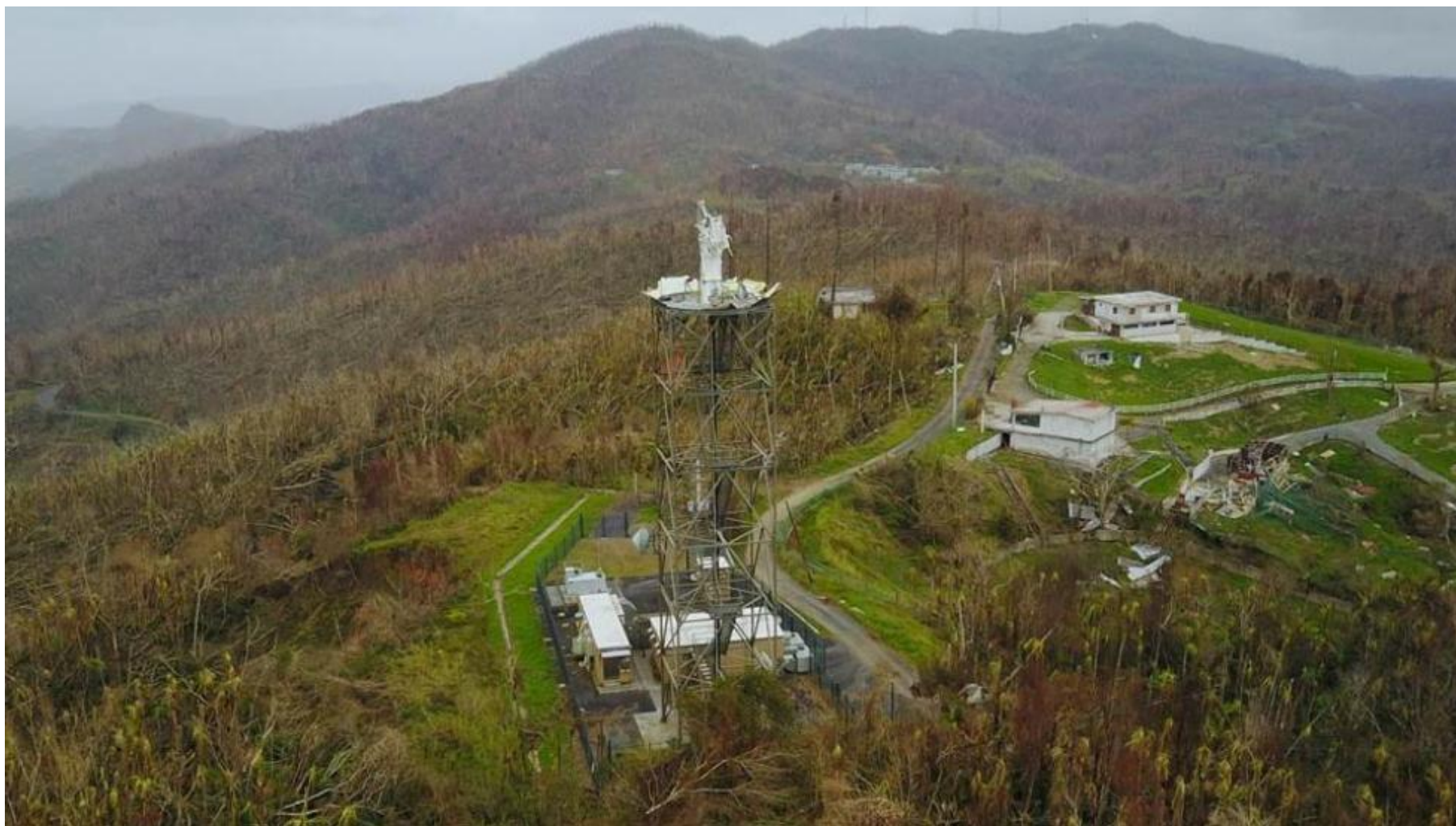
Figure 10. The remnants of the San Juan WSR-88D radar after its destruction by Hurricane Maria. Photo credit: WFO San Juan.
